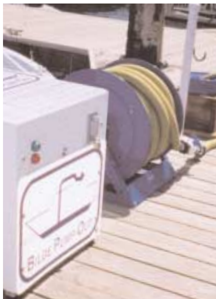
Clearly labeled bilge pumpout facility
